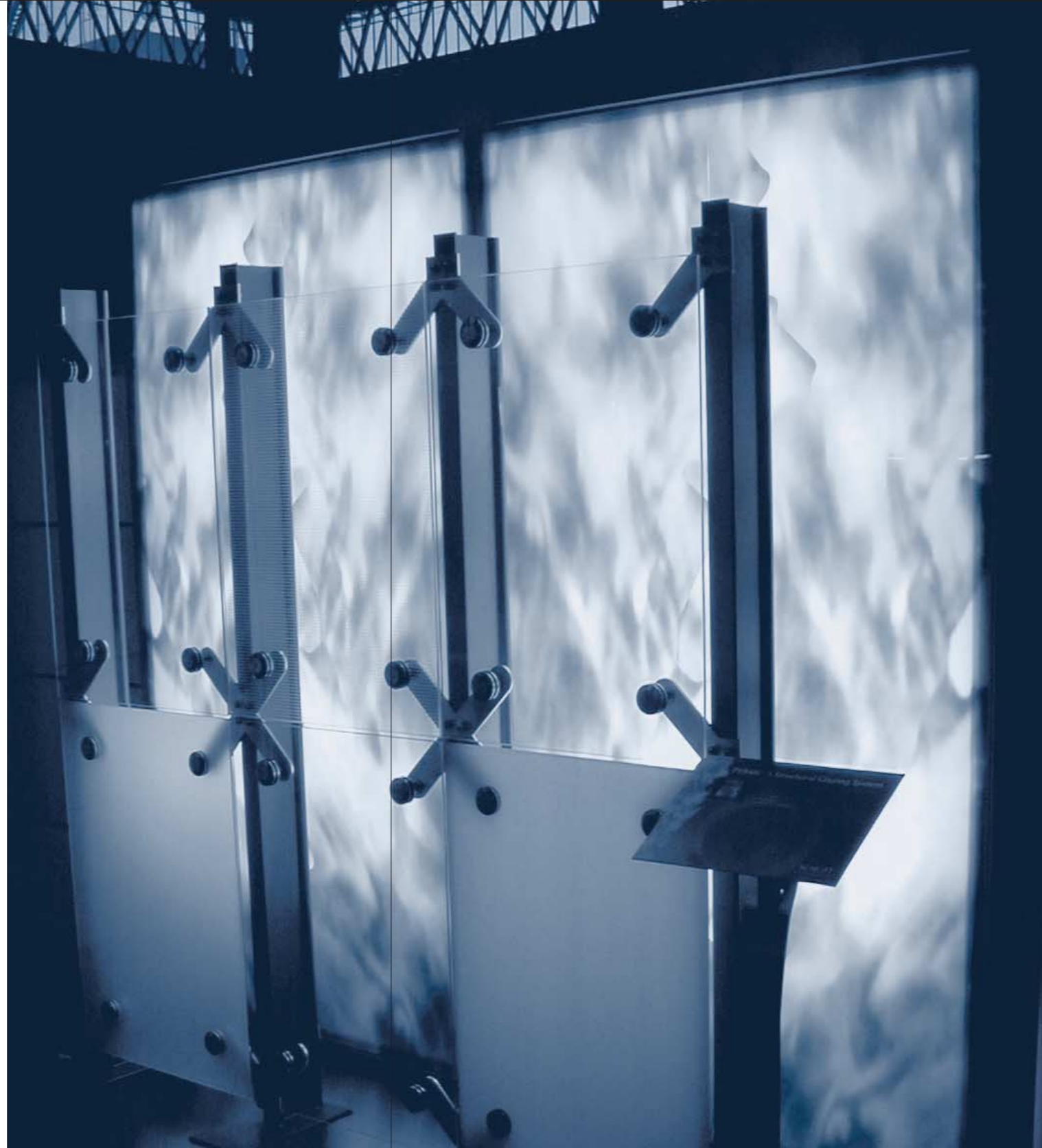
These T-Profiles are typical of the support steelwork.
