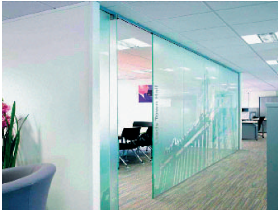
Toughened glass is up to four or five times stronger than annealed glass and laminates made from it are exceptionally strong.
